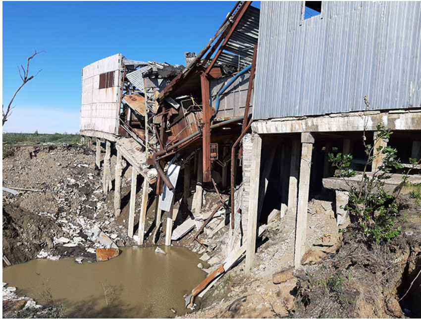
Figure 4: Thawed Permafrost Collapses Building [4]
