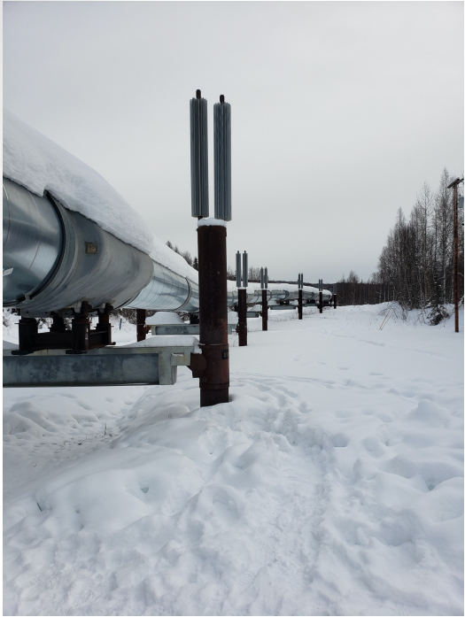
Figure 3: Alaska Pipeline Thermosyphons
